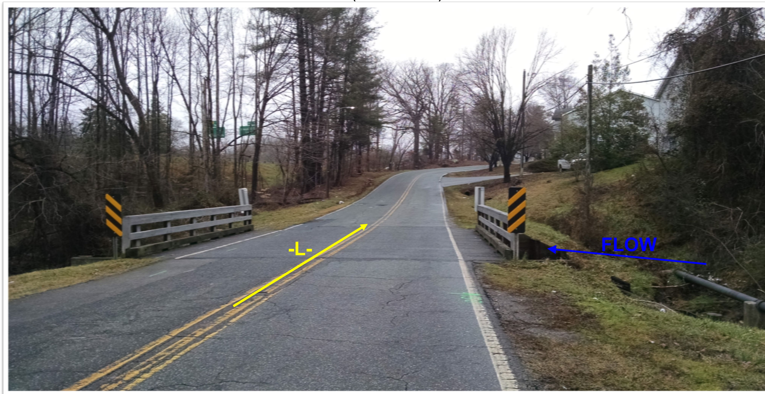
Looking Upstation from Sta. 12+00, -L-
